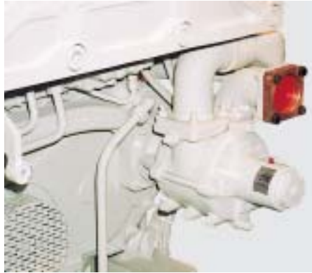
Installation of centrifugal pump KB
